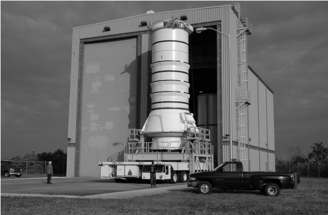
Figure No. E-47. The right aft booster, comprised of the aft skirt and aft motor segment, rolls out of a Surge Building at the RPSF for transfer to the VAB, where it will be stacked for Discovery , STS-121, January 23, 2006.
